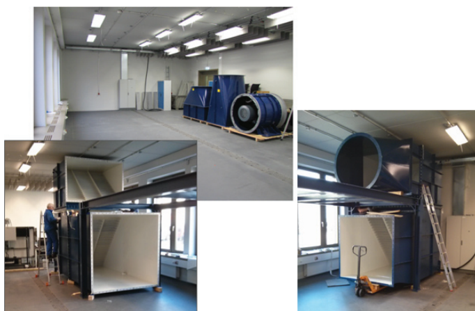
Figure 6: Corner regions with the baffles are installed in countercurrent directions in the laboratory; ventilator region is prepared to be installed at top of the frame structure.
