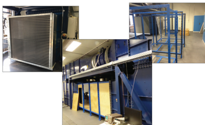
Figure 7: Construction of the nozzle region and connection in between the corner regions; material of nozzle regions is PMMA and wood for a higher flexibility; left: heat exchanger installation downstream of test section.
